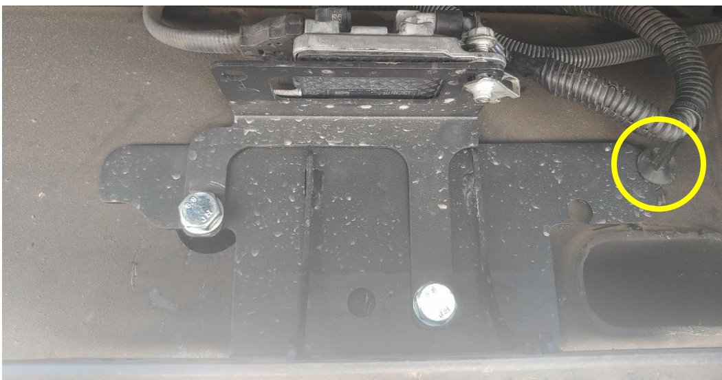
Figure 16- Compressor Bracket Installation 2, Diesel
