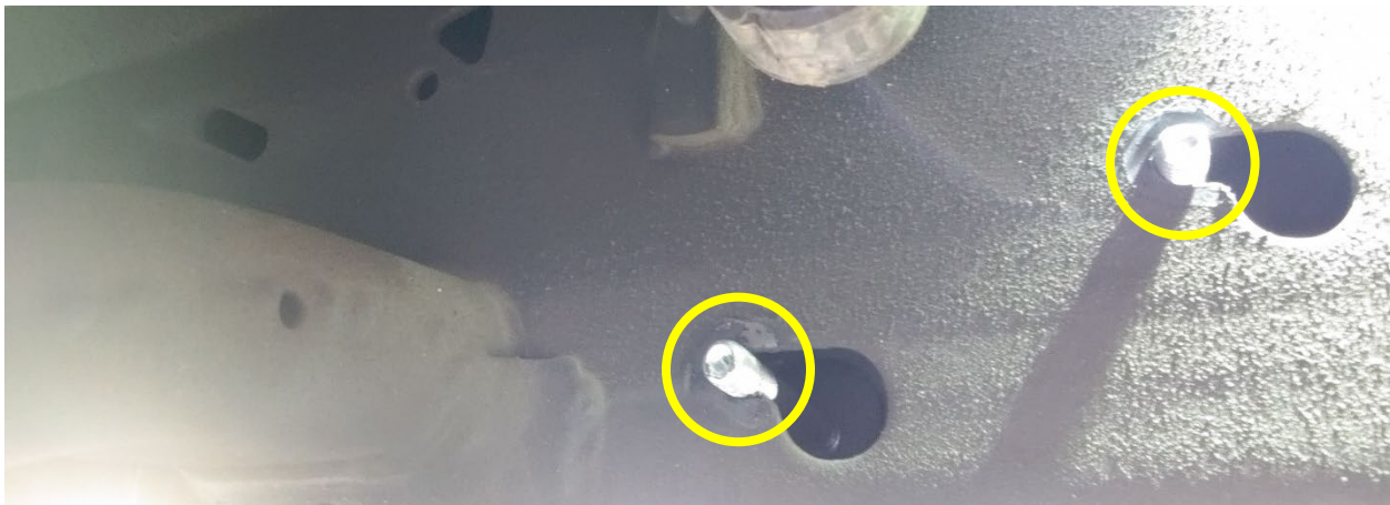
Figure 12- Compressor Bracket Installation, Inside Frame Rail
