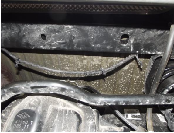
Photo 1 – Horizontal beam with wiring harness clips removed
