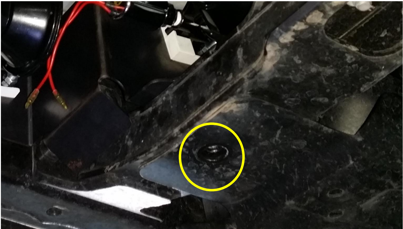
Figure 9 - Factory Gas Tank Skid Plate Bolt
