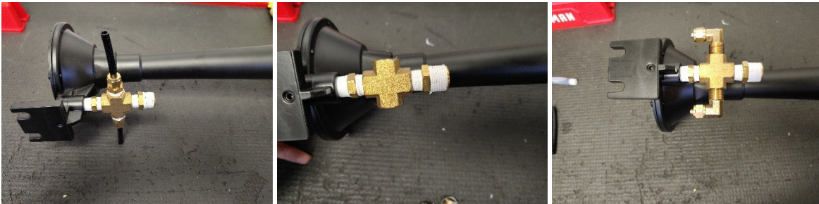
Figure 8- Medium Horn Fitting Replacement
