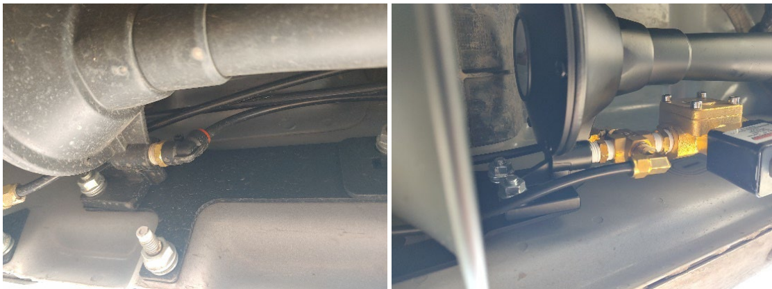
Figure 29- Small & Medium Horn Installation
