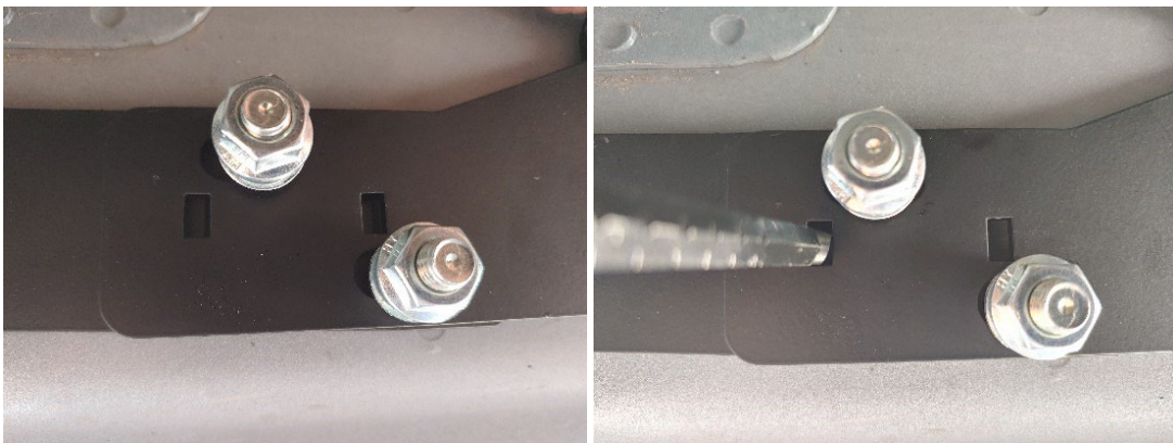
Figure 27- Dual Horn Bracket Installation 2
