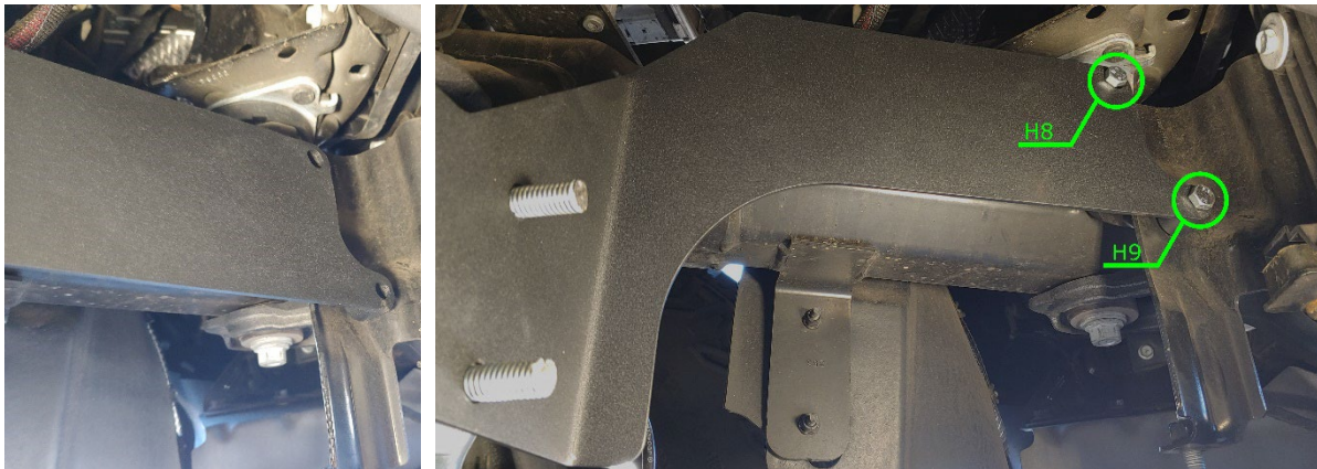
Figure 25- Primary Tank Bracket Installation 2, Step 11
