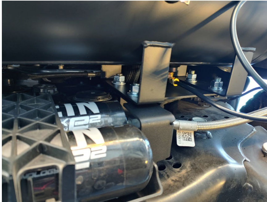
Figure 26- Tank, Installed System Plumbing
