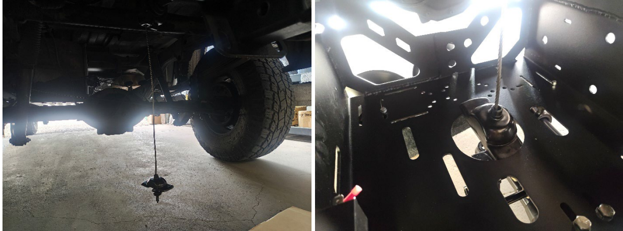
Figure 19- USTL On-Vehicle Install #1
