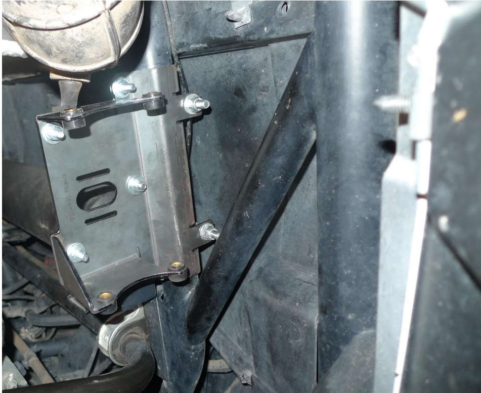
Figure 15 - Air Compressor Bracket Installed on Frame
