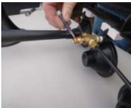
Preparing to install the solenoid
