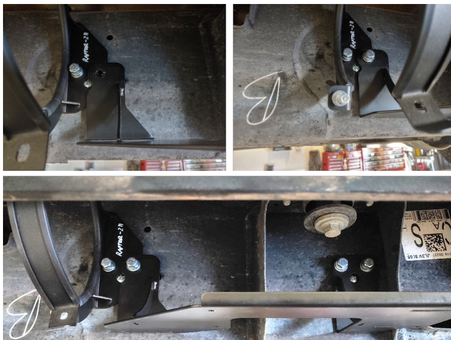
Figure 12- Compressor & Front Tank Bracket Installed
